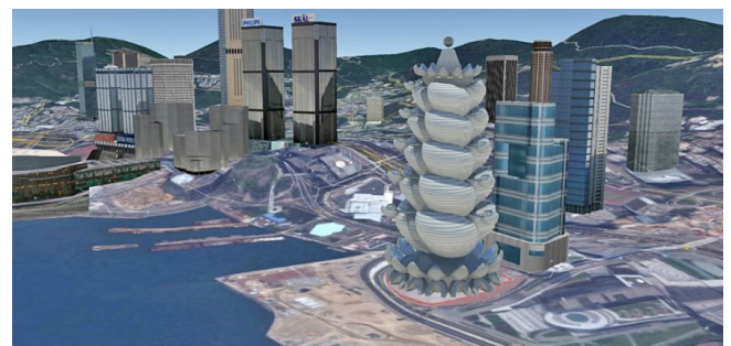
Fig. 3. Arcology Skyscraper, Hong Kong. Articulation of five similar facade elements, equipped with water spheres, located in carrying spoons vibration damping in an earthquake
