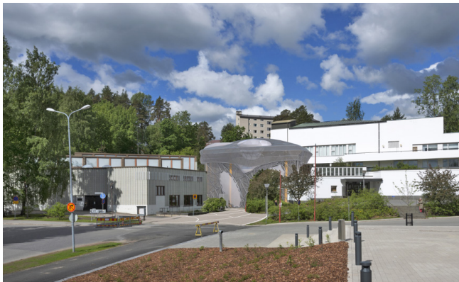
Fig. 1. General view of the extension between the two museums
