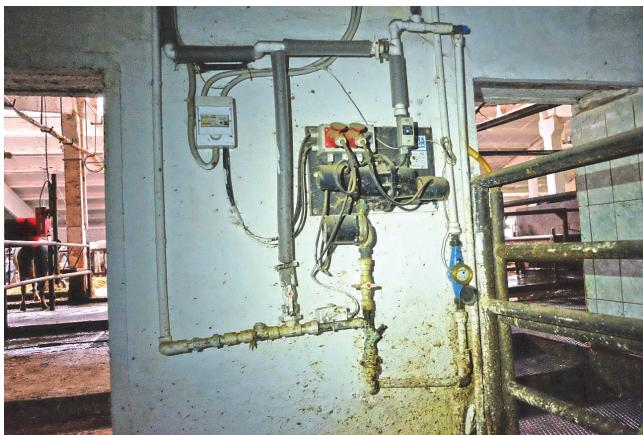
**Fig. 5. Installation of the circulating heating water in drinking bowls**
