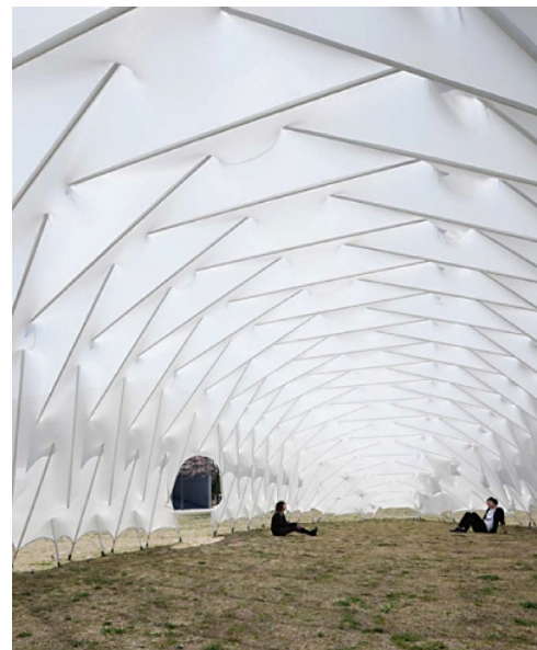
Fig. 16. Space formed under the stretched membrane of tensegrity-structure suitable for placement of refrigerators for fruits and vegetables for medical purposes (2016a.secure.ifai.com)
